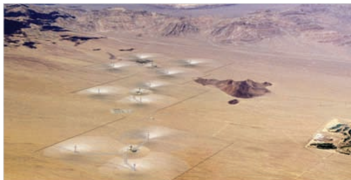
400 MW Solar Power Complex Being Developed By BrightSource
